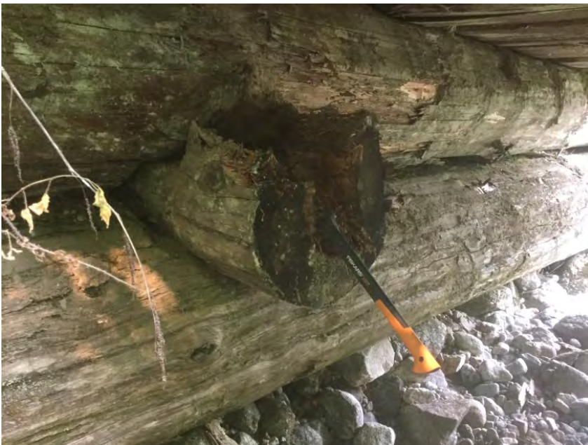
Tieback condition on left abutment
