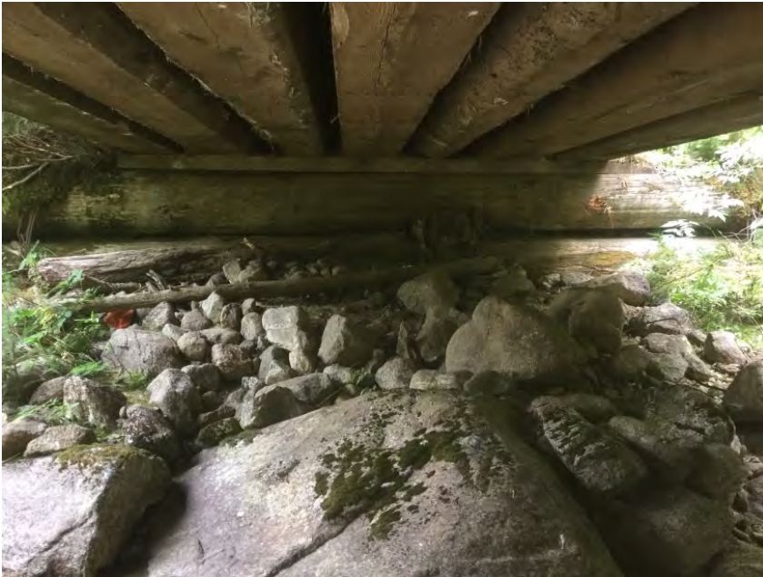
Right Bank Abutment when facing downstream
