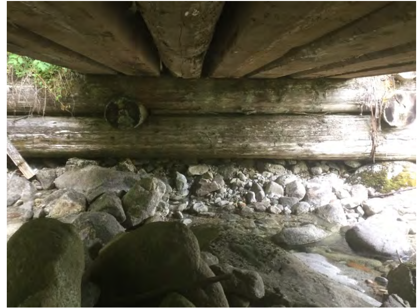
Left Bank Abutment when facing downstream
