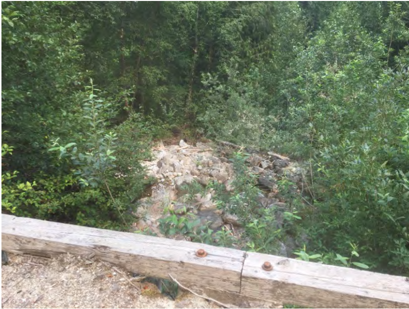
Looking downstream from deck
